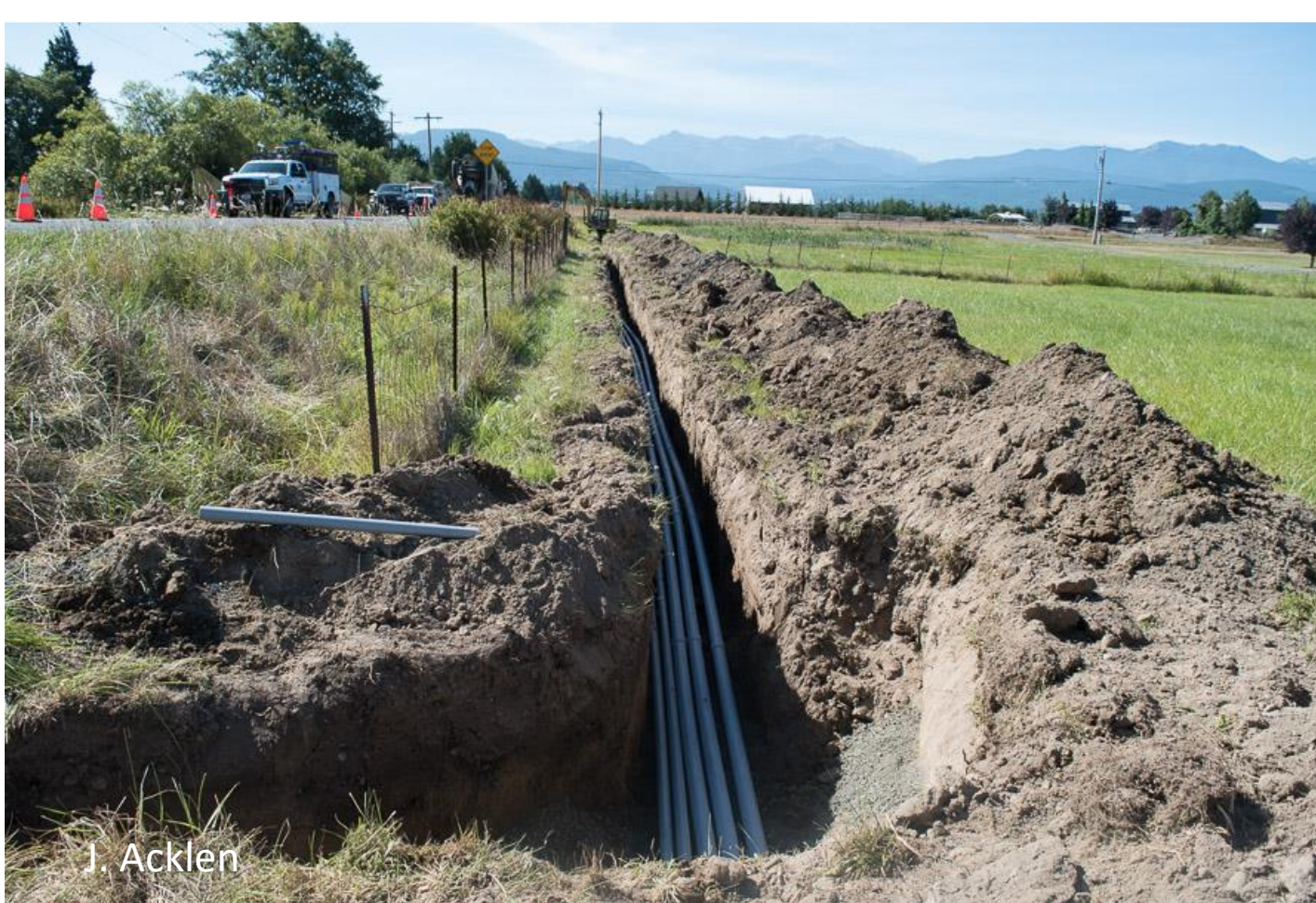
Conduit in utility trench along Kirner Rd
