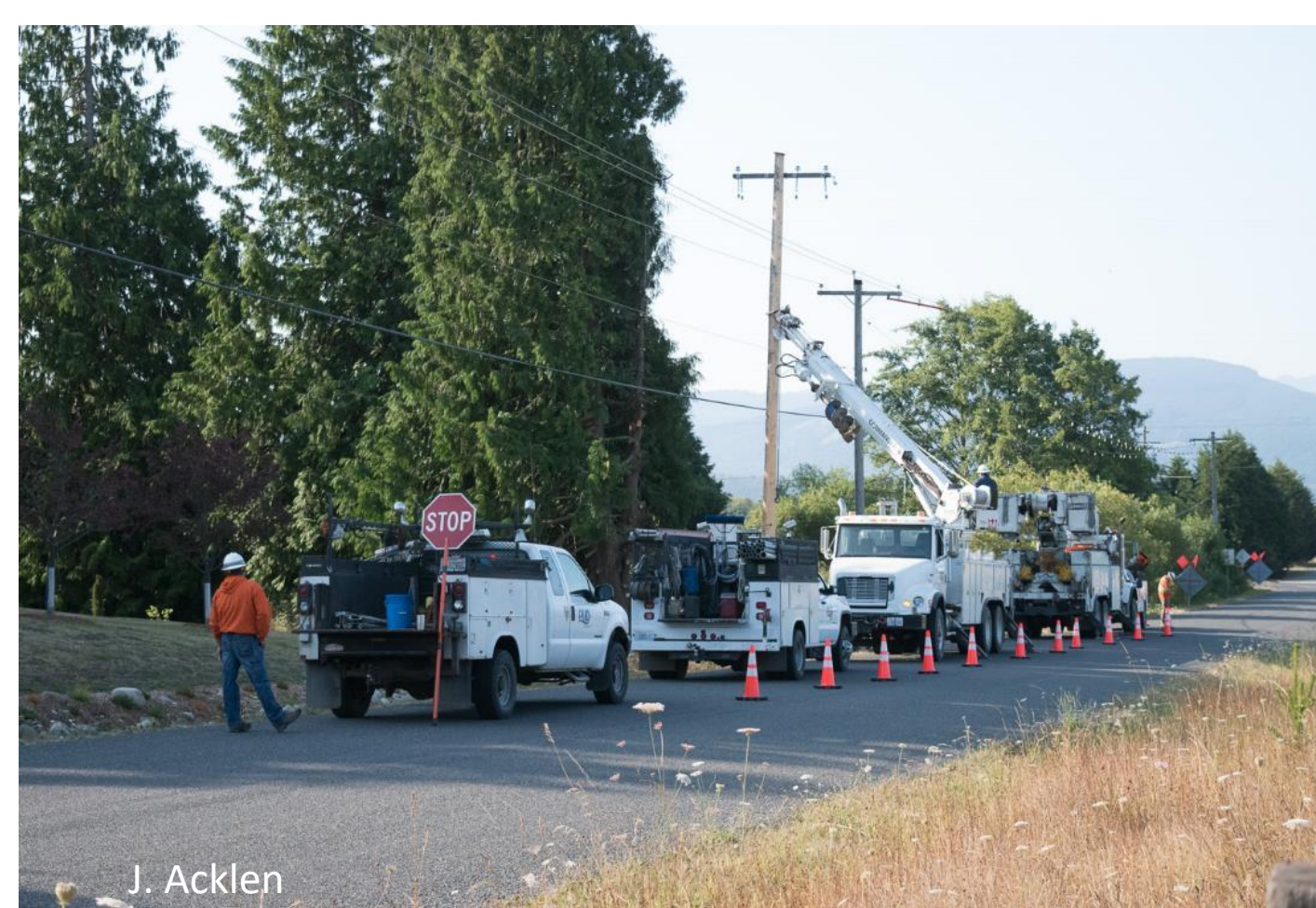
PUD installs a new riser at Kirner Pond
