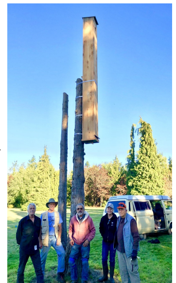
Finished Installation and Team Photo by Jennifer Margison
