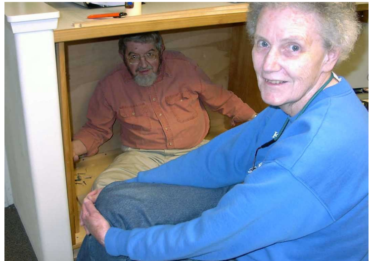
Virginia & Weldon Clark installing River Center audio-visual system
