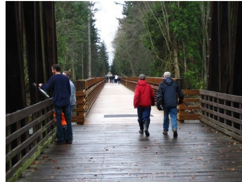
New Bridge Trestle Photo by Tom Butler
